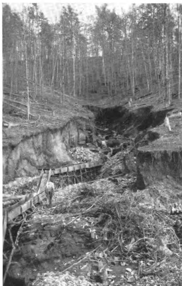
A. BEGINNING OF A HYDRAULIC CUT IN SAPROLITE, TOPABRI MINE, LUMPKIN COUNTY, GA. Photograph by W. D. Johnston, Jr.
