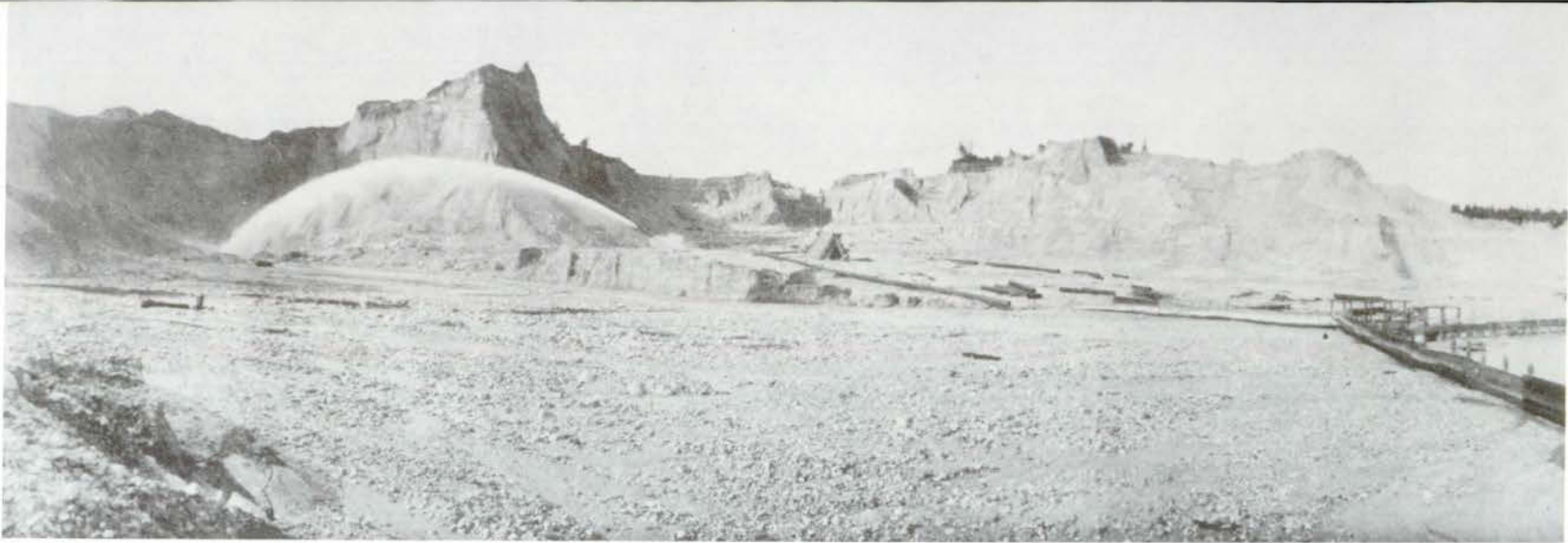
Figure 2. Hydraulic Mining of Surface Gravel in North Columbia Pit. (Circa 1880)
