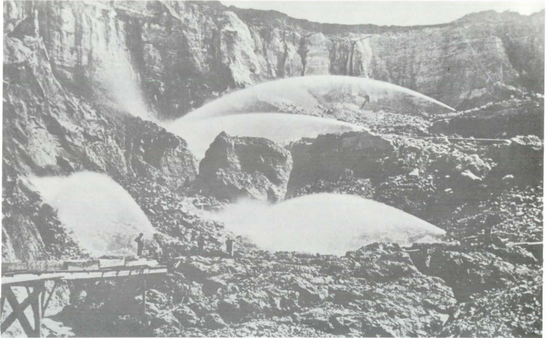
Figure 1. Hydraulic Mining Operations in Malakoff Diggings Pit. (Circa 1880)
