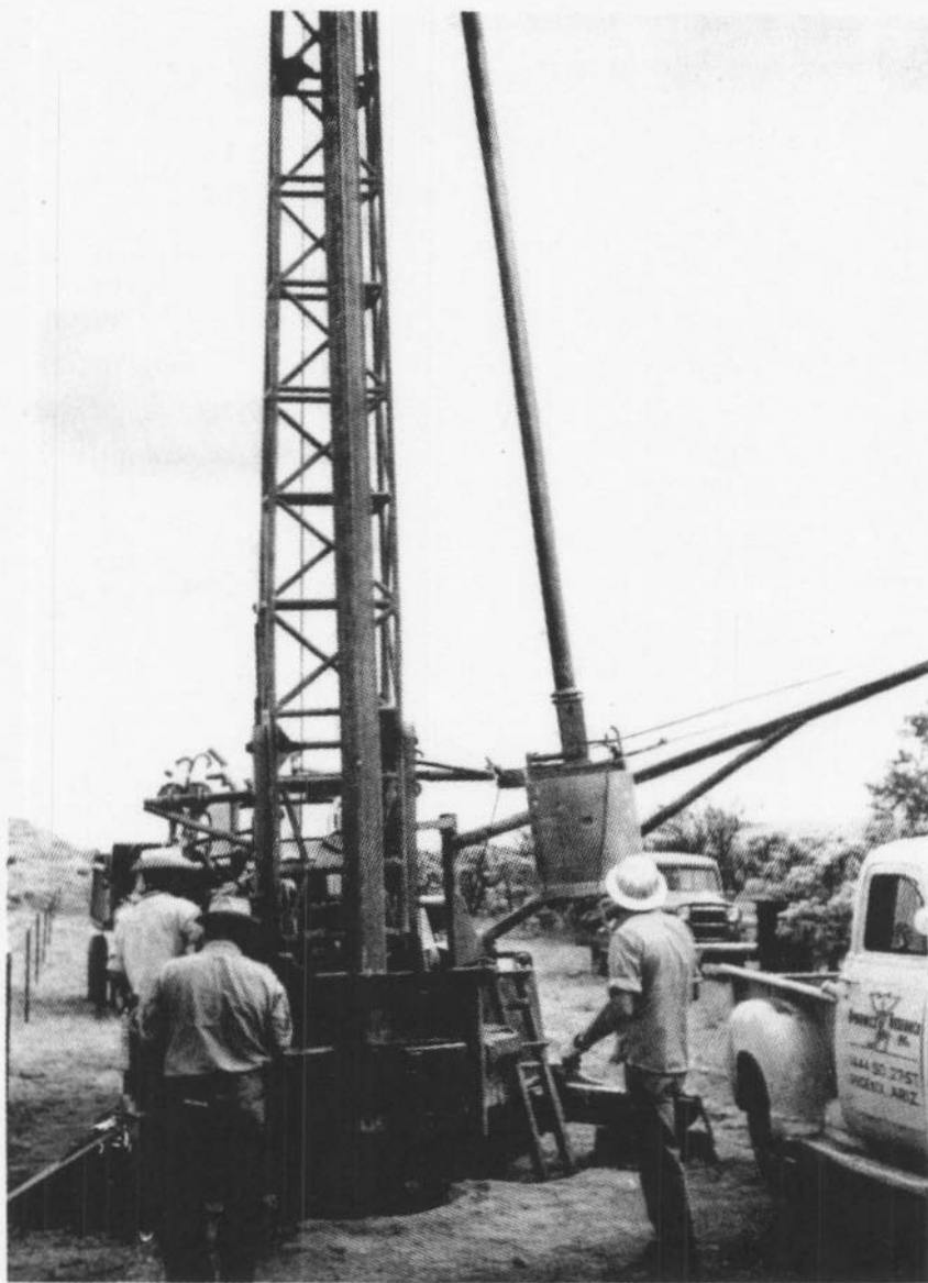
FIGURE 4. — Rotary bucket drill making a 24-inch diameter hole in desert placer material. The average drilling rate for 90 foot holes was about 70 feet per shift. Progress was slowed by the presence of numerous hard, caliche-cemented layers.
