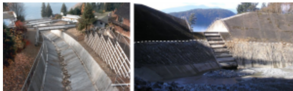
Figure 15.22 Two strategies for mitigating debris flows on the Sea-to-Sky Highway. Left: A concrete-lined channel on Alberta Creek allows debris to flow quickly through to the ocean. Right: A debris-flow catchment basin on Charles Creek. In 2010, a debris flow filled the basin to the level of the dotted white line. [SE]
