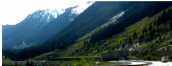
Figure 15.21 A snow avalanche shelter on the Coquihalla Highway. The expected path of the avalanche is the steep un-treed slope above. [SE]
