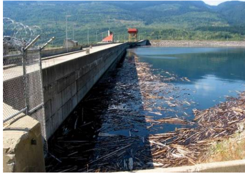
Revelstoke Dam and Revelstoke Lake on the Columbia River at Revelstoke, BC [SE]
