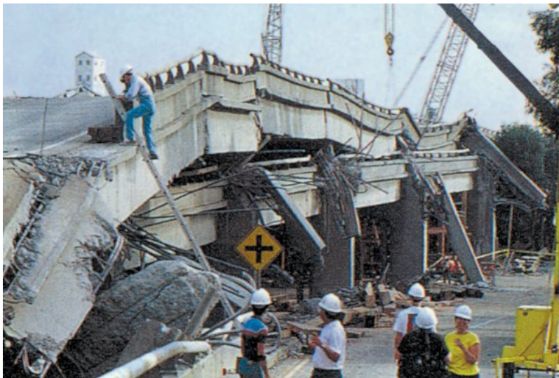
Figure 11.17 A part of the Cypress Freeway in Oakland California that collapsed during the 1989 Loma Prieta earthquake. [from: http://upload.wikimedia.org/wikipedia/commons/9/91/Cypress_collapsed.jpg ]
