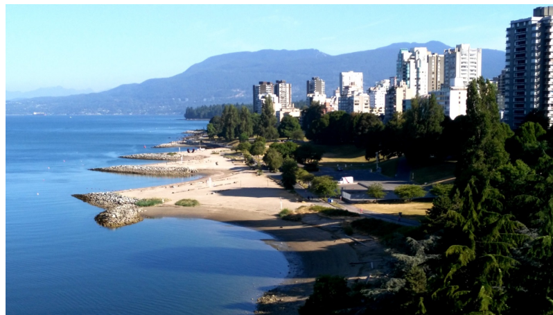
Figure 17.30 Photograph of the impact of breakwaters on beach development at Sunset Beach, Vancouver [by Isaac Earle, used with permission]
