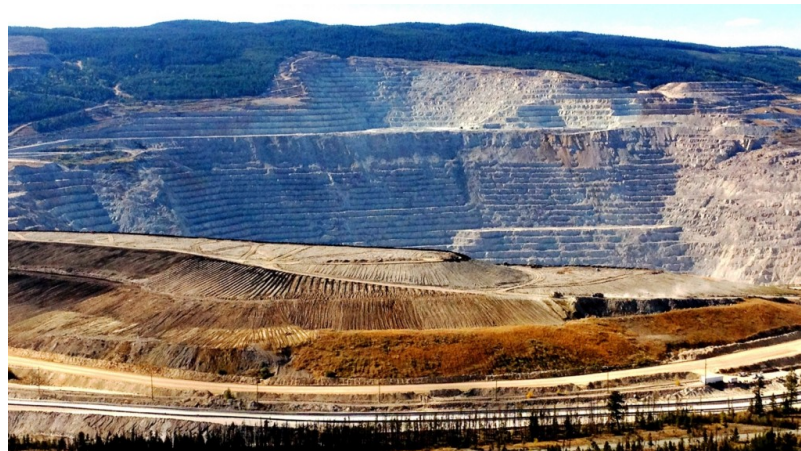
Figure 20.1 The open pit (background) and waste-rock piles (middle) of the Highland Valley Copper Mine at Logan Lake, British Columbia [Photo by Russell Hartlaub, used with permission]
