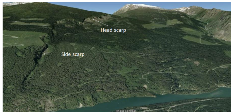
Figure 15.9 The Downie Slide, a sackung, on the shore of the Revelstoke Reservoir (above the Revelstoke Dam). The head scarp is visible at the top and a side-scarp along the left side. [from Google Earth]
