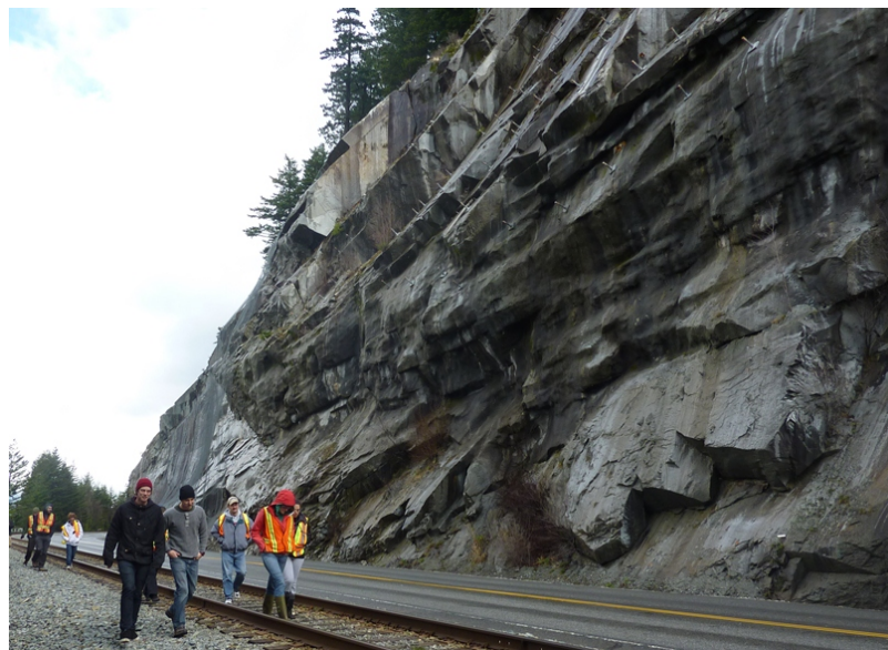
Figure 15.10 Site of the 2008 rock slide at Porteau Cove. Notice the prominent fracture set parallel to the surface of the slope. The slope has been stabilized with rock bolts (top) and holes have been drilled into the rock to improve drainage (one is visible in the lower right). Risk to passing vehicles from rock fall has been reduced by hanging mesh curtains (background). [SE photo 2012]
