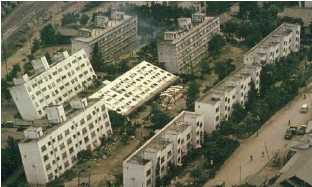
Figure 11.22 Collapsed apartment buildings in the Niigata area of Japan. The material beneath the buildings was liquefied to varying degrees by the 1964 earthquake. http://en.wikipedia.org/wiki/1964_Niigata_earthquake#/media/File:Liquefaction_at_Niigata.JPG
